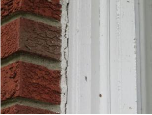
Failing caulk
